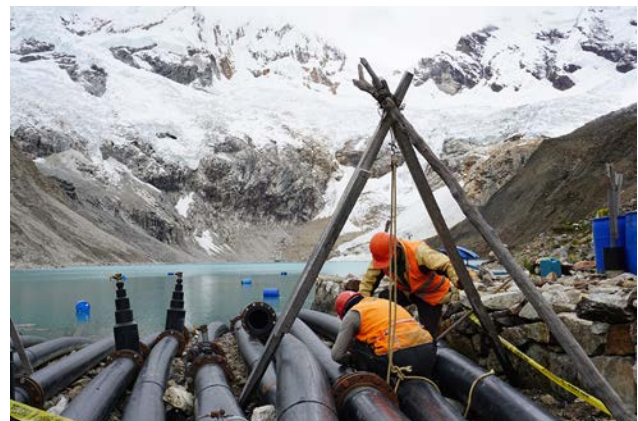
Figure 7. The Palcacocha Glacier lake (Peru) is drained using siphons to avoid Glacier Lake Outburst Floods (GLOF) (courtesy Christian Huggel (Switzerland))
